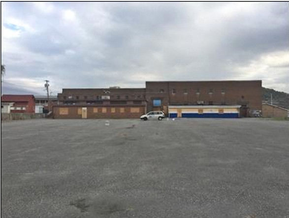
Old Keyser High School Building Photo 3.jpg
