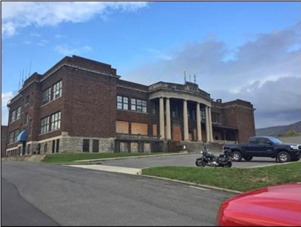
Old Keyser High School Building Photo 1.jpg
