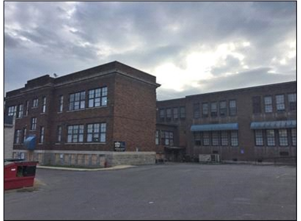
Old Keyser High School Building Photo 2.jpg
